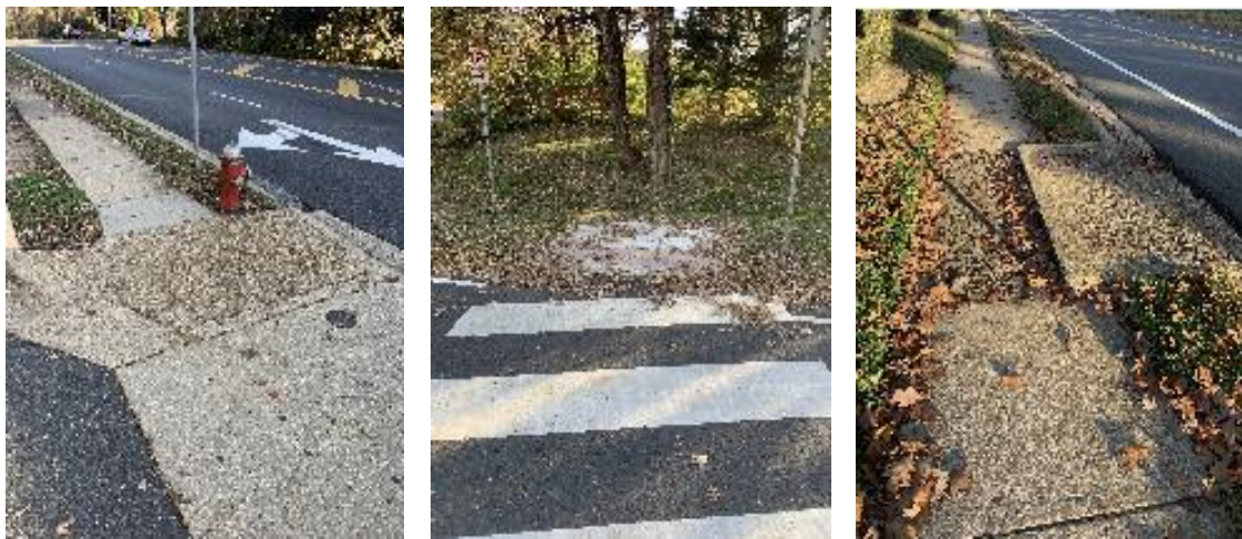
Figure 5. Examples of (a.) Lack of Truncated Dome, (b.) Missing Section/Connection, and (c.) Protruding Object along public right of ways Woodburn Rd and Tobin Rd.
